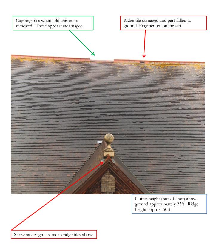
General area of roof damaged is ridge (not possible to photograph from ground level)
