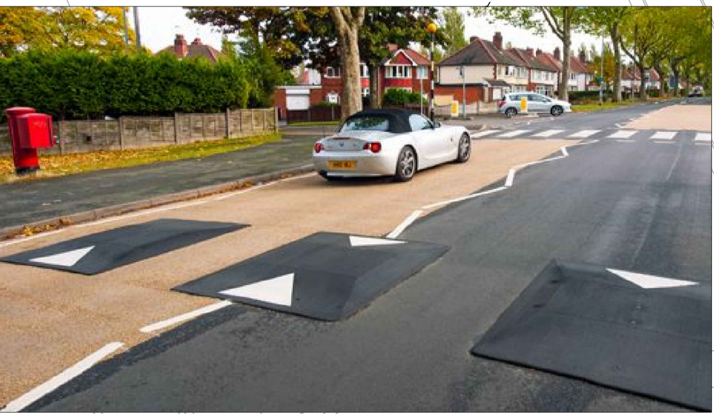
Example of a 3 speed cushion arrangement used to maintain slower traffic speeds.
