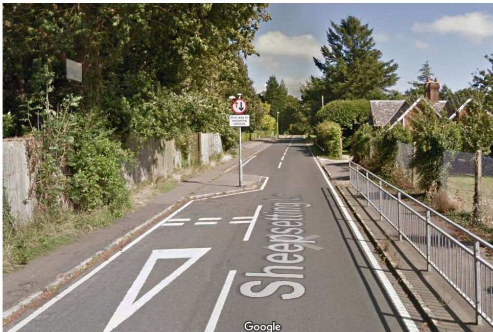
Figure 4.3: - Typical horizontal calming feature - simple priority working.
