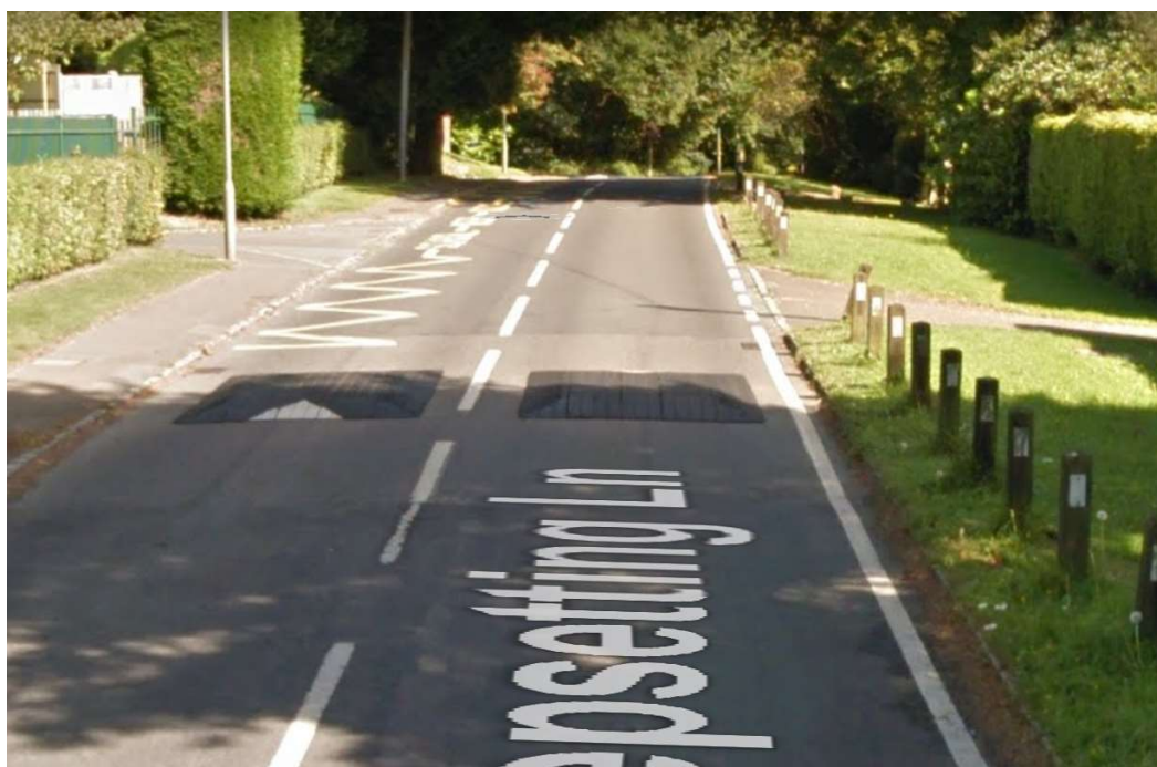
Figure 4.1: - Example of a vertical calming feature – speed cushion
